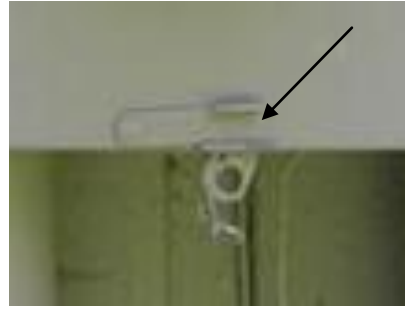
The loop on the electric box.
