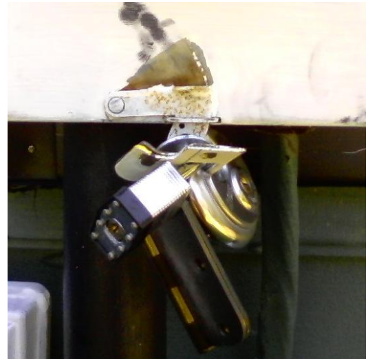
Pic 3. Box with shielded shackle lock thru loop and additional locks and hardware attached thru the lock's loop. You can't really see the shackle lock here (it's on the right), just the nuts, locks, etc threaded through the loop. Note that there is still easy access to the loop for the meter, which an installer can cut with a hacksaw. They are destroying your property if they do so (the meter housing belongs to you), but they will sometimes do it, and it is possible that DTE will make this a policy. This is why you should take the next step and use a cage, bar, or angle bracket.
