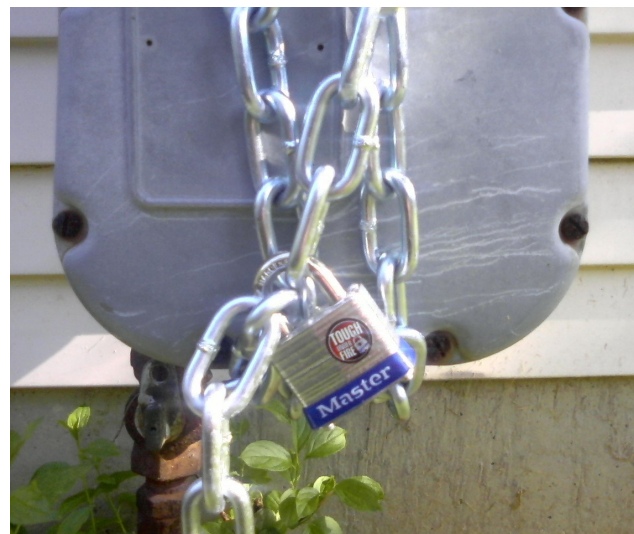
Close-up of lock on gas meter.
